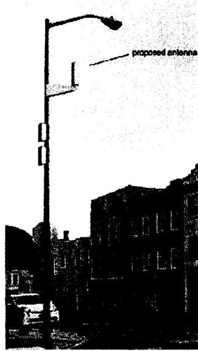
Figure 19.53.030-b: Side-arm mounted antennas are not permitted.
