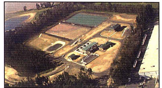
Aerial View of Wastewater Plant
