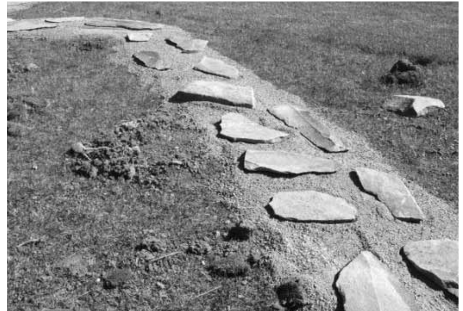
Installing hardscaping prior to sheet mulching
