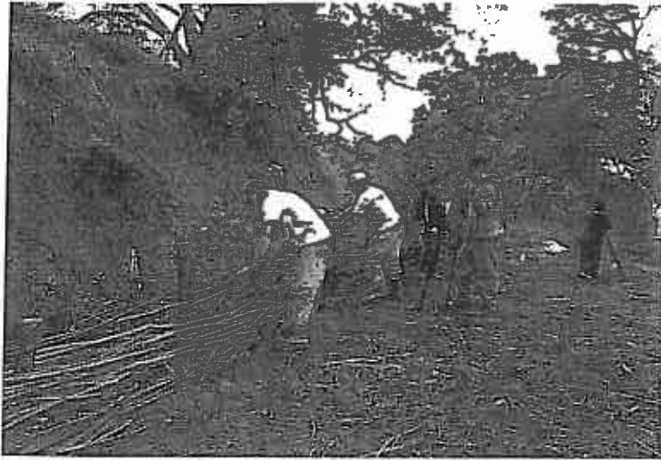
Photo 2- 5. Willow Revetment- Willow revetments are a very effective, low cost means of controlling stream bank erosion. On most sites, they can be built without the need for heavy equipment, just able-bodied labor. Collection of dormant plant material should be conducted as near to the planting site as possible. Trained volunteer crews, the California Conservation Corp., or private restoration firms are capable of performing the work, depending on the complexity of treatment needed.
