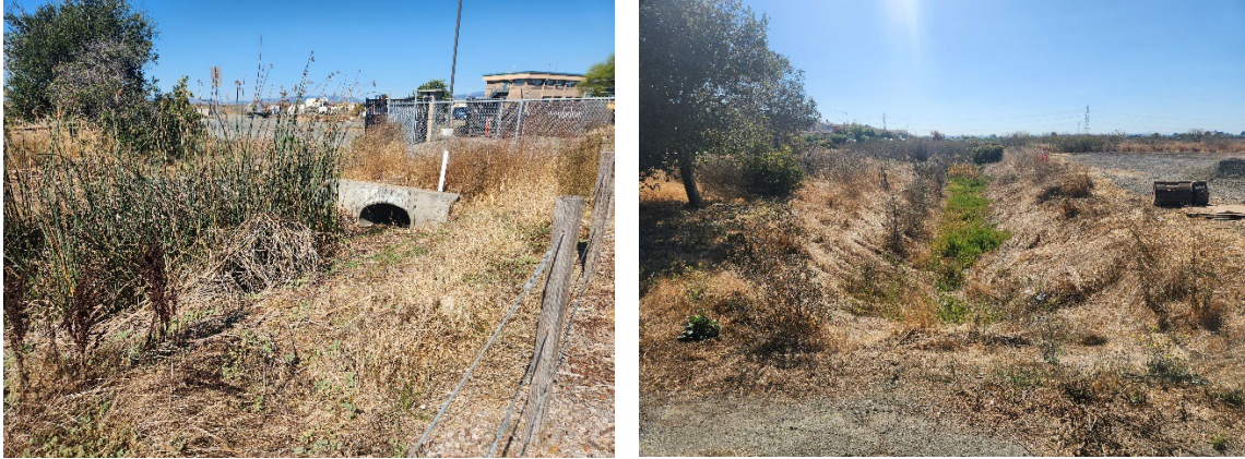
Figure 6 Storm Drain Outfall and Drainage Swale at Corporation Yard
